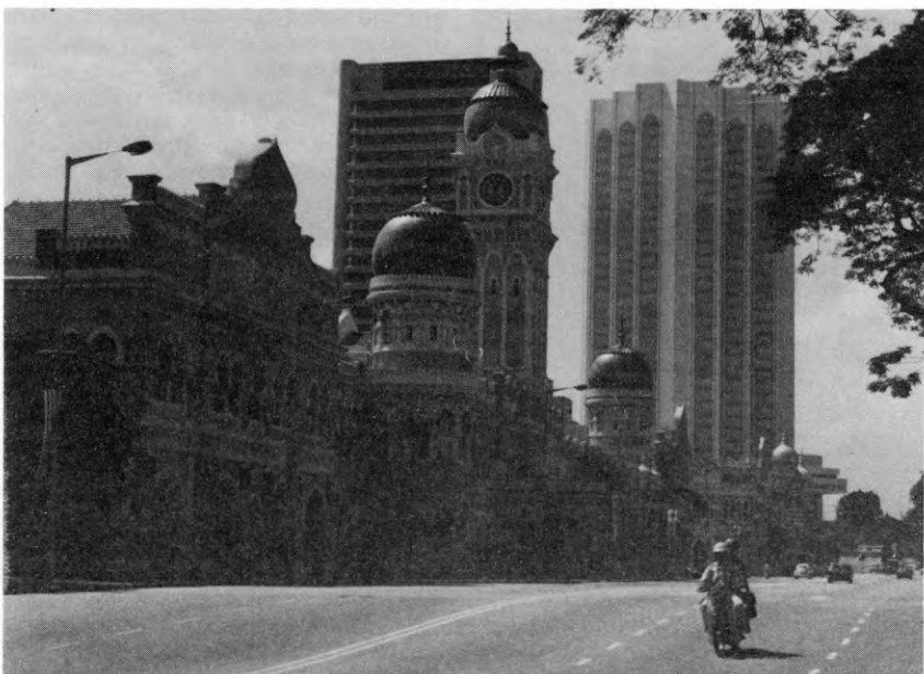
• The old and the new in K.L. architecture. In the foreground are the law courts which date back to British Administration days.
