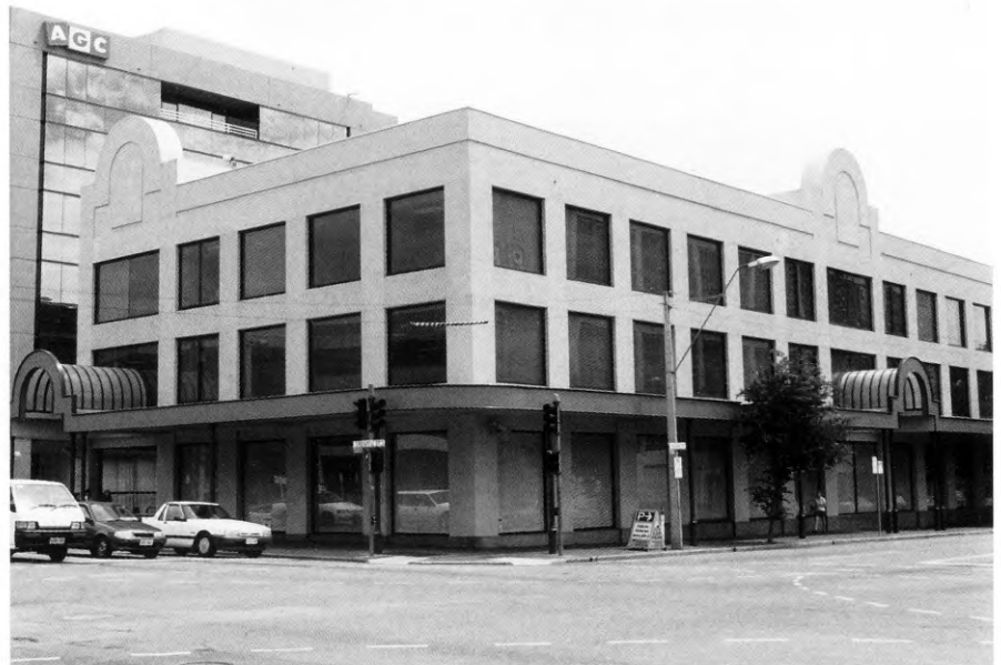
Central Region's head office is now located within Adelaide's central business district.
