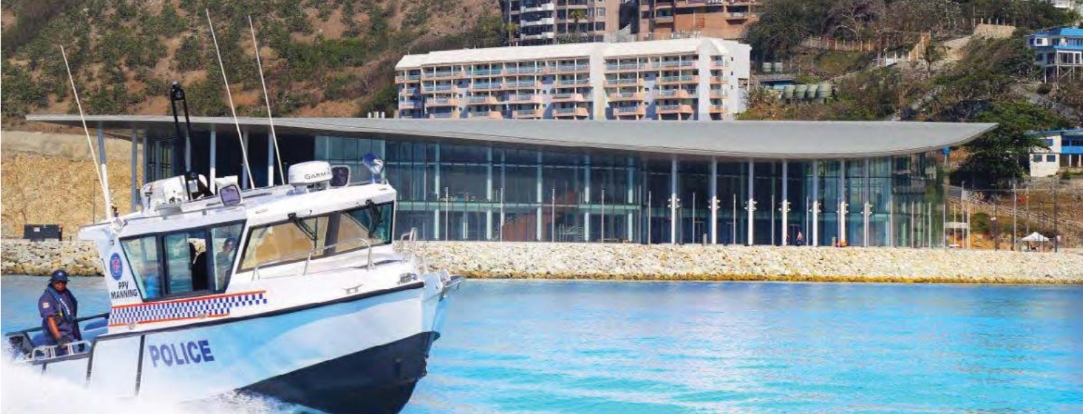
A Royal Papua New Guinea Constabulary water policing vessel keeps APEC Haus secure from the sea.
