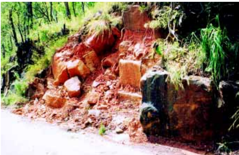
This small landslide on the Paluma Road, north of Townsville, killed a woms during Tropical Cyclone Justin in March 1997
