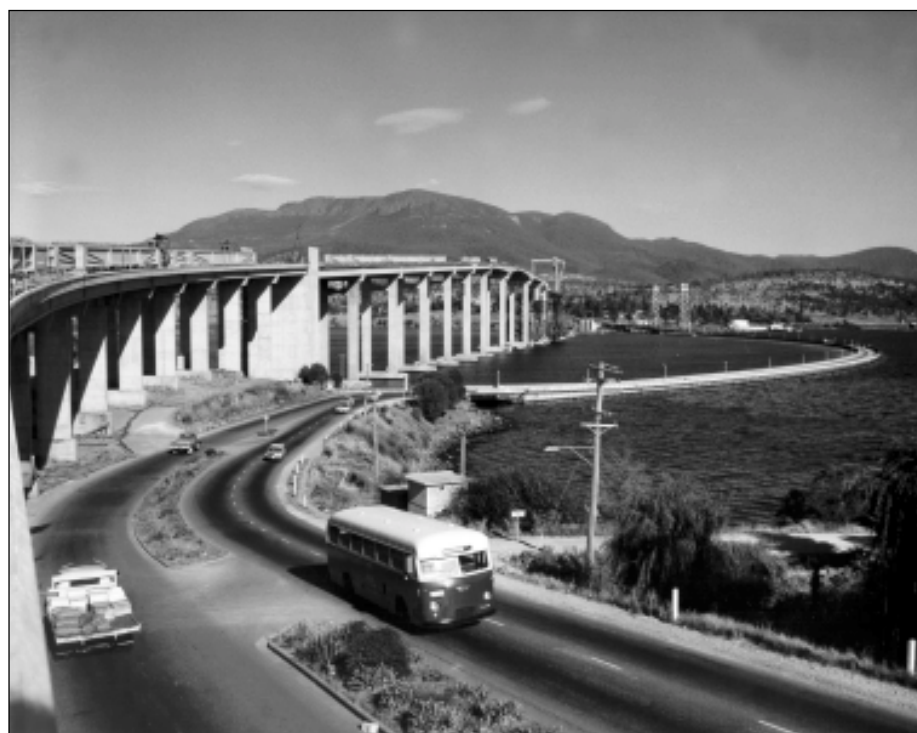
Figure 2 –Tasman Bridge during construction and floating arch bridge
