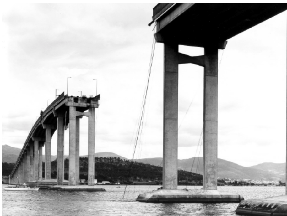
Figure 3 – Tasman Bridge, 6 January 1975
