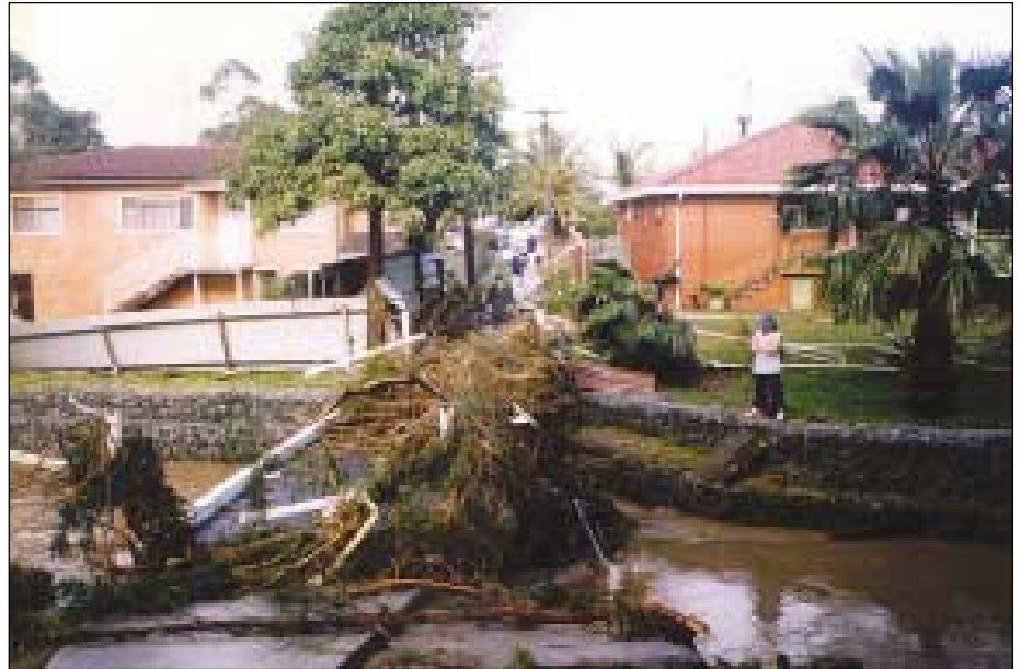
The City of Wollongong, in NSW, received disastrous flooding in August 1998. Excessive runoff from the adjacent escarpment produced significant inundation problems on the numerous small creeks and watercourses that traverse the established urban areas of the city. In particular, debris in the form of rocks and boulders, vegetation, cars and other household items caused blockage of numerous culverts and small bridges. This debris exacerbated inundation problems. Recent studies have identified that many of the city culverts were virtually fully blocked during the flood. This debris problem, and the additional inundation resulting from it, placed unexpected demands on the local SES personnel.
