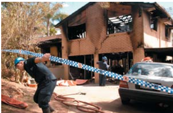
Two children were trapped, and subsequently died in this house fire.
