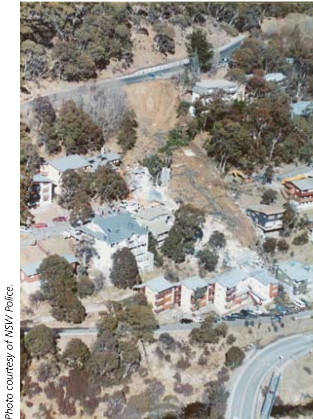
This landslide of 30 July 1997 at Thredbo claimed 18 lives as a consequence of the destruction of two ski lodges by a failure of the road embankment fill of the Alpine Way.
