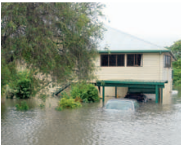
An estimated 200 homes experienced disruption to power, telecommunications and an overflow to sewerage systems.
