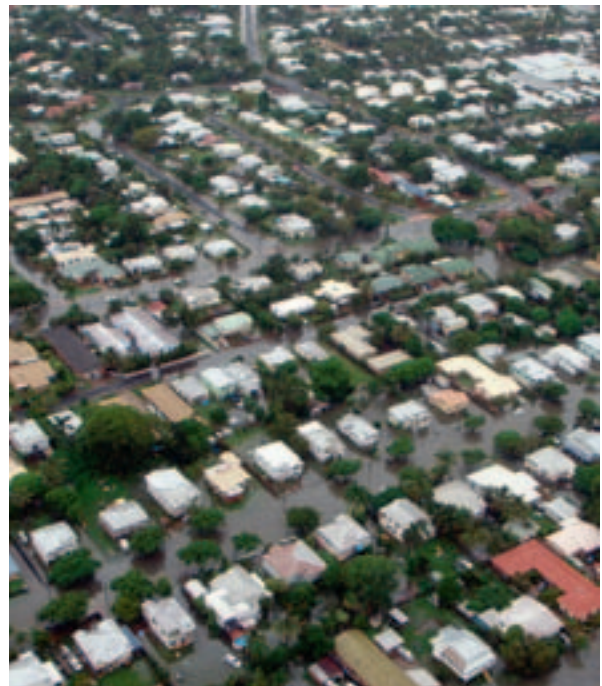
A rebuild of parts of the city was required after the floods.
