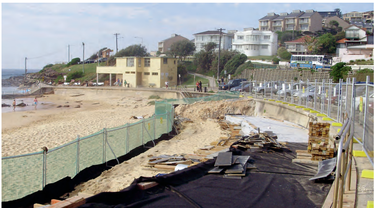
Reconstruction work on Collaroy Beach, Sydney, Australia.
