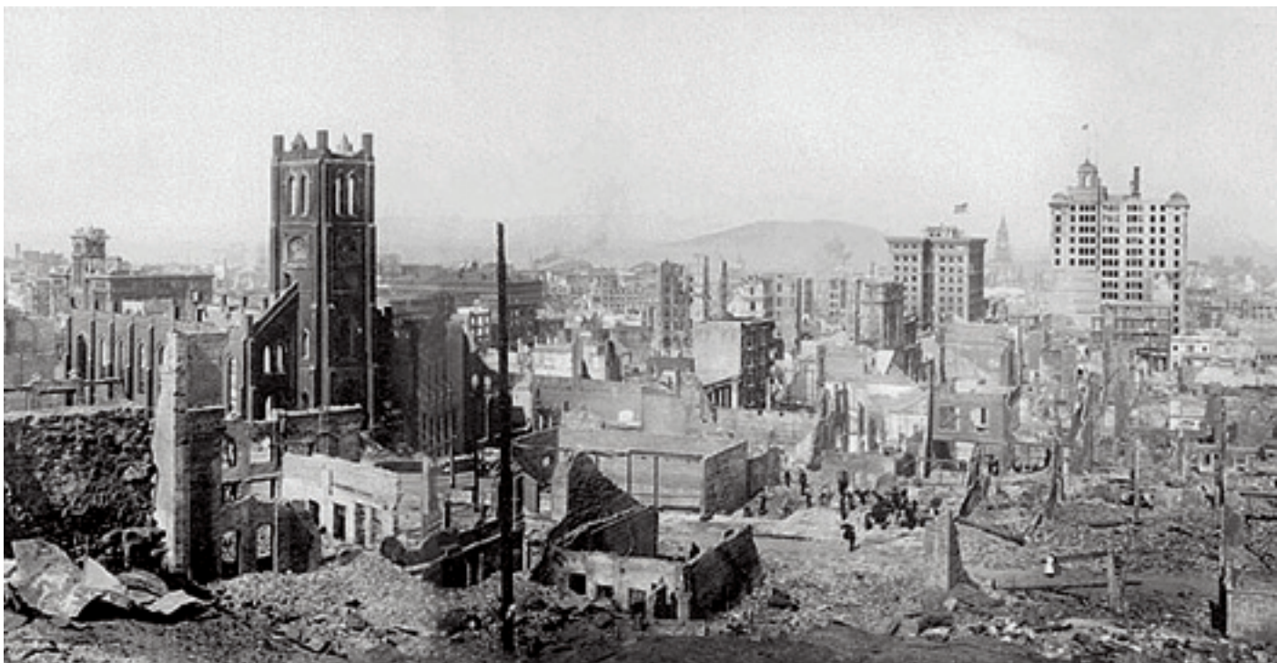
San Francisco earthquake.
