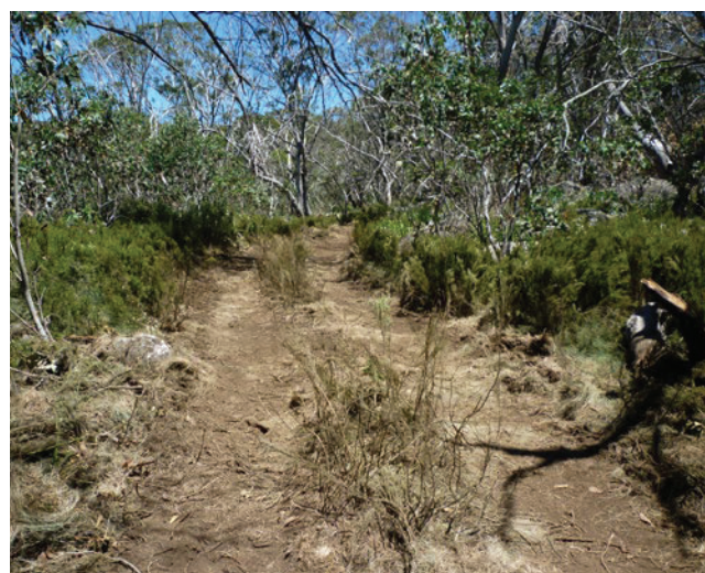
The northern containment line after the fire. The bulldozers were instructed by the Divisional Commander to retain topsoil to aid rehabilitation. The D4 removed the shrub layer while the bigger blade on the D6 was used to remove branches from the Snow Gums ( Eucalyptus pauciflora ).
