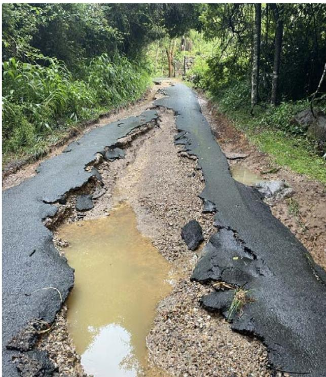
Receding flood waters exposed extensive damage to large sections of local roads.
