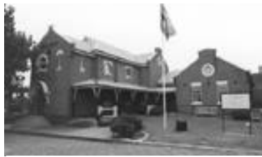
Cowra Court House
