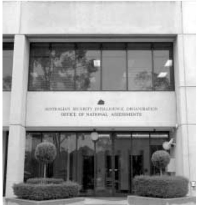
The ASIO building part of the Russell Defence complex. Photo: Michael Jones / News Image Library
