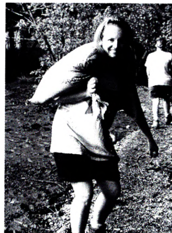
CHRISTY CARRYING MATERIALS IN PREPARATION FOR 3 SOLID DAYS LAYING CEMENT
