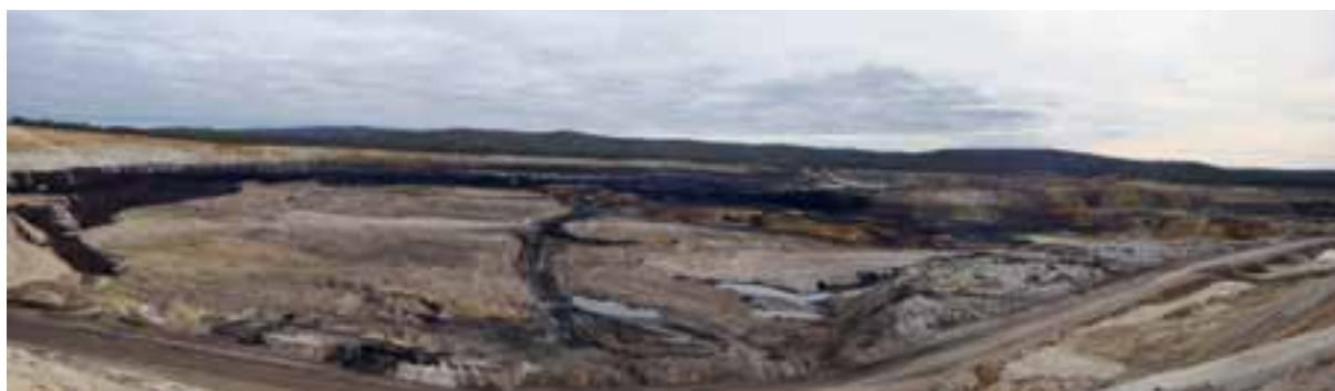
Figure 7. Panoramic photograph of the Anglesea mine showing the progressive coverage of the pit floor by overburden as at 29 July 2015. 158
